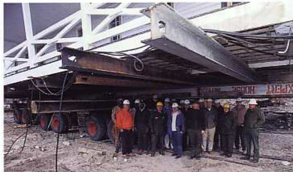
BENEATH THE DOUBLE KEEPER'S QUARTERS: Paul Cloyd (center, blue coat) and co-workers pause during a progress meeting.
