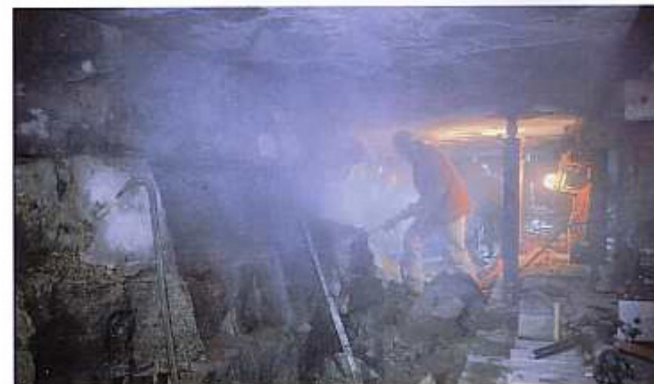
DOWN UNDER: A worker removes granite from under the lighthouse.
